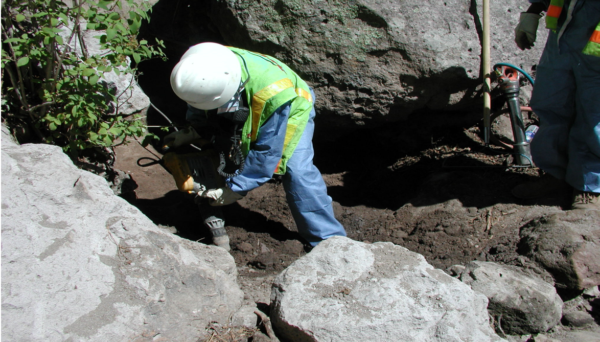
Removal of contaminated media from the drainage below the SWMU 01-001(f) outfall
