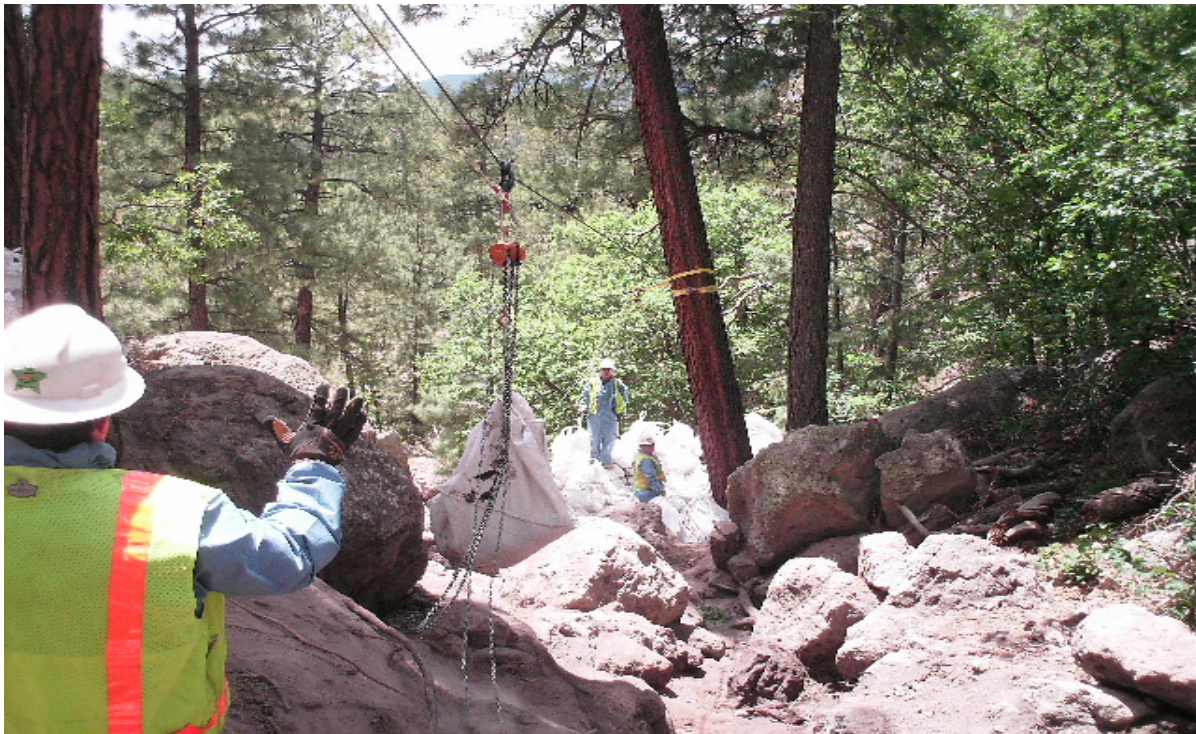
Transfer of waste bags from hillside drainage to canyon bottom via zip line
