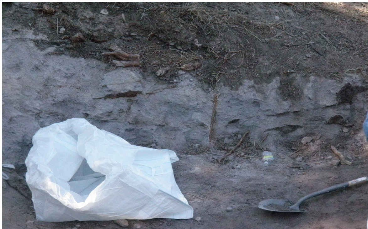
Shovel removal and packaging of contaminated media within the SWMU 01-001(f) outfall area
