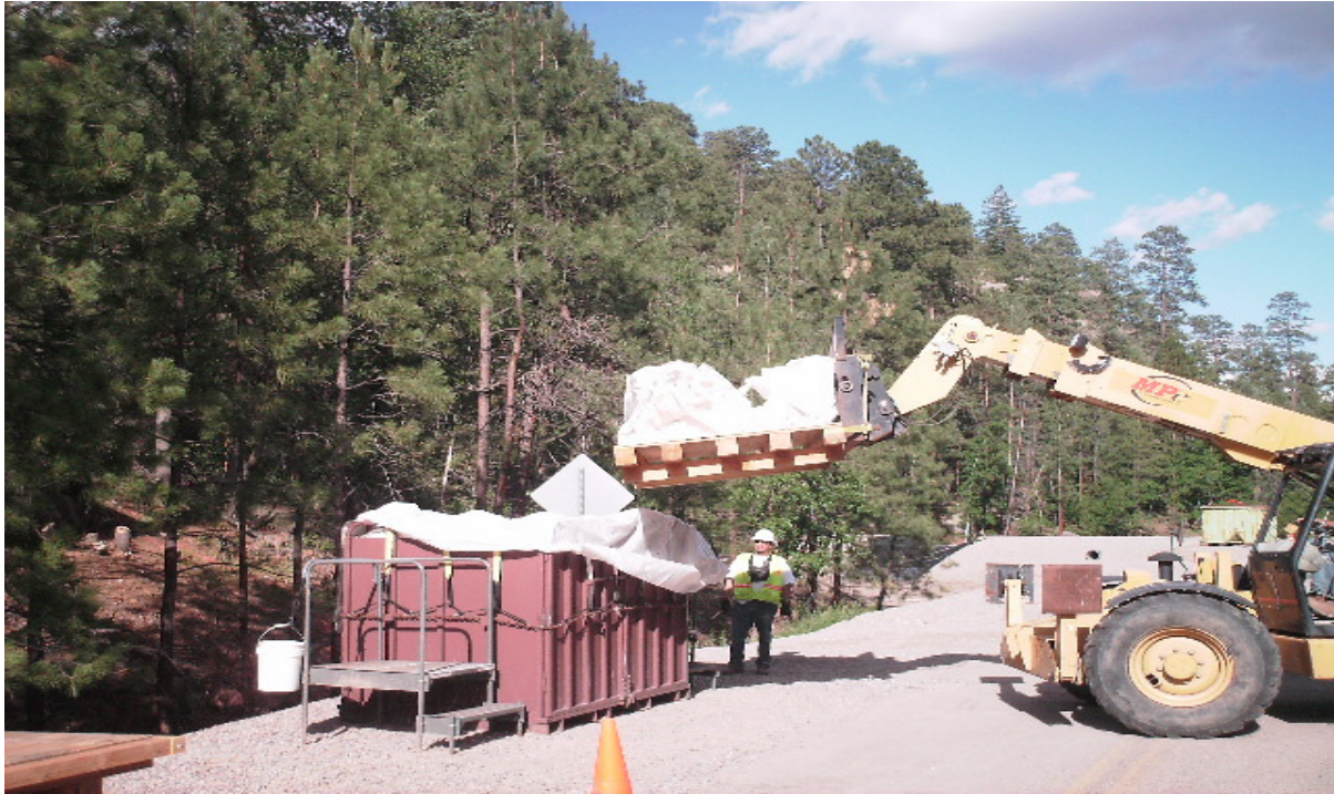
Bags of excavated media being loaded into waste box in the bottom of Los Alamos Canyon
