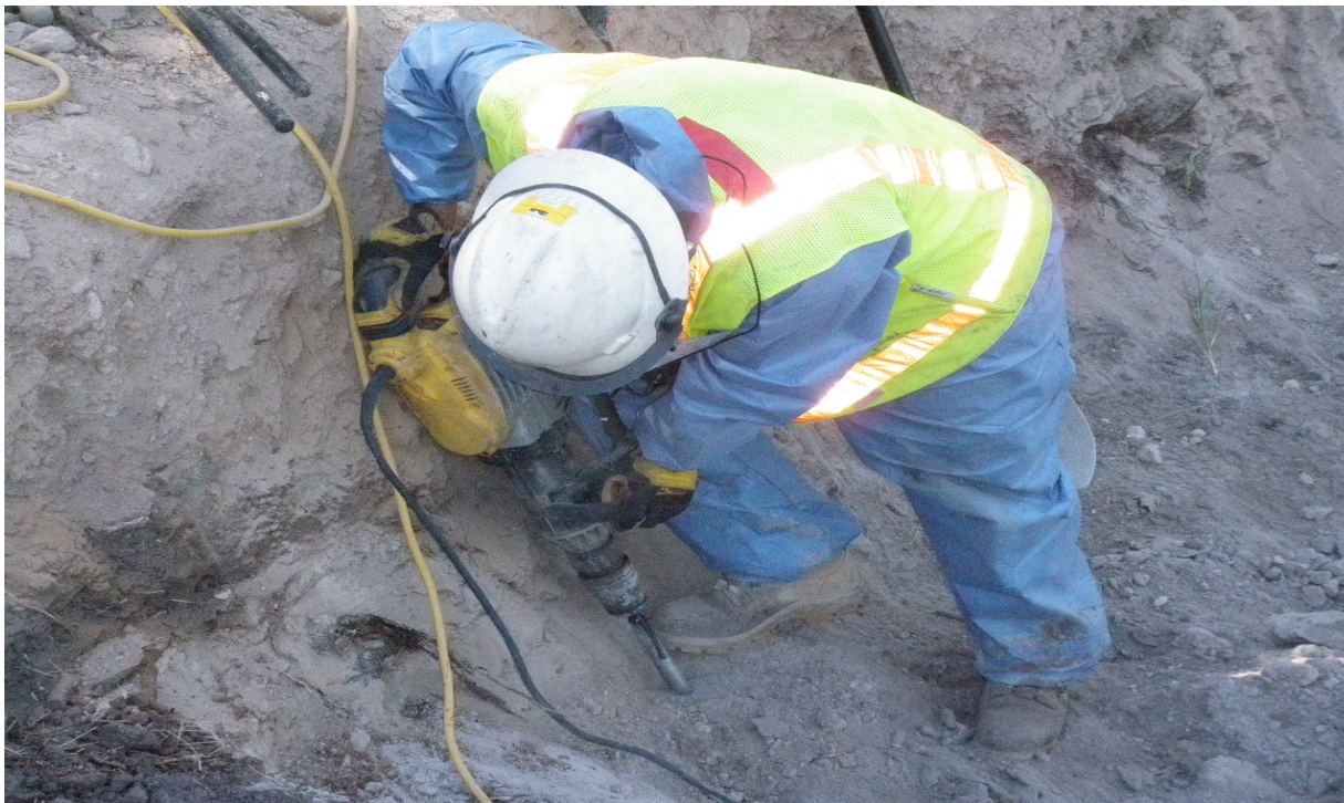
Use of air hammers to remove contaminated media from drainage below the SWMU 01-001(f) outfall
