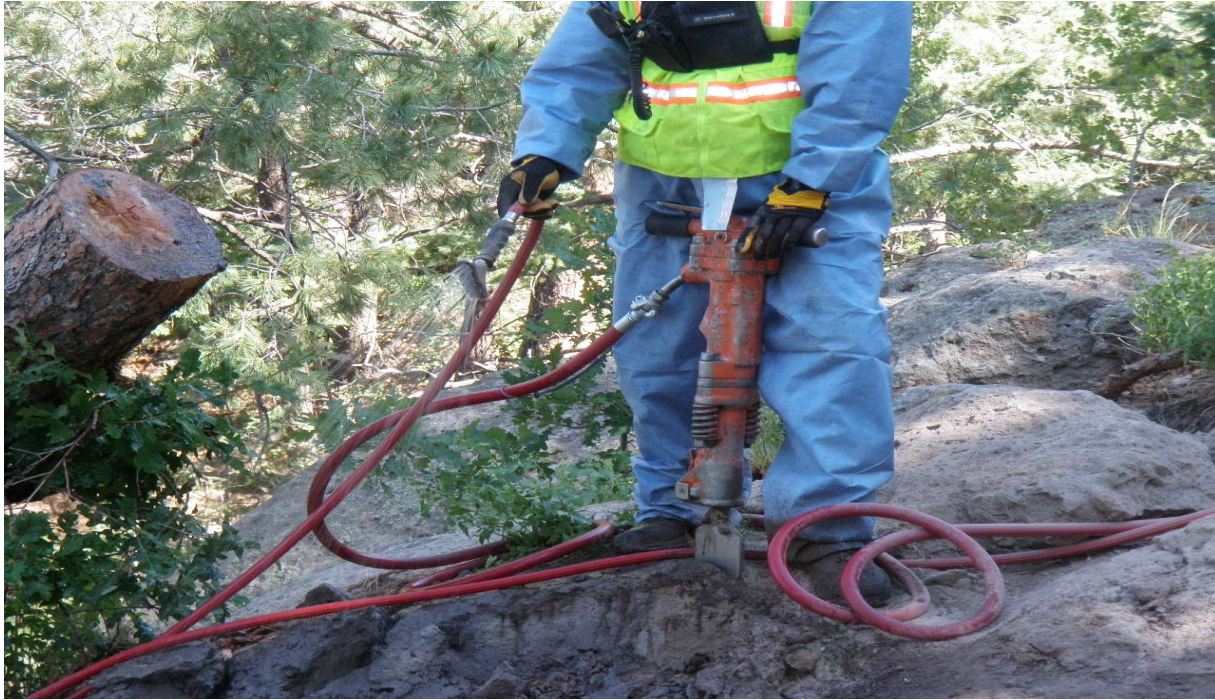
Use of air hammers to remove contaminated media from drainage below the SWMU 01-001(f) outfall
