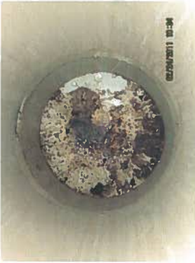
West basin, west inspection Pipe. (2/24/2011)
