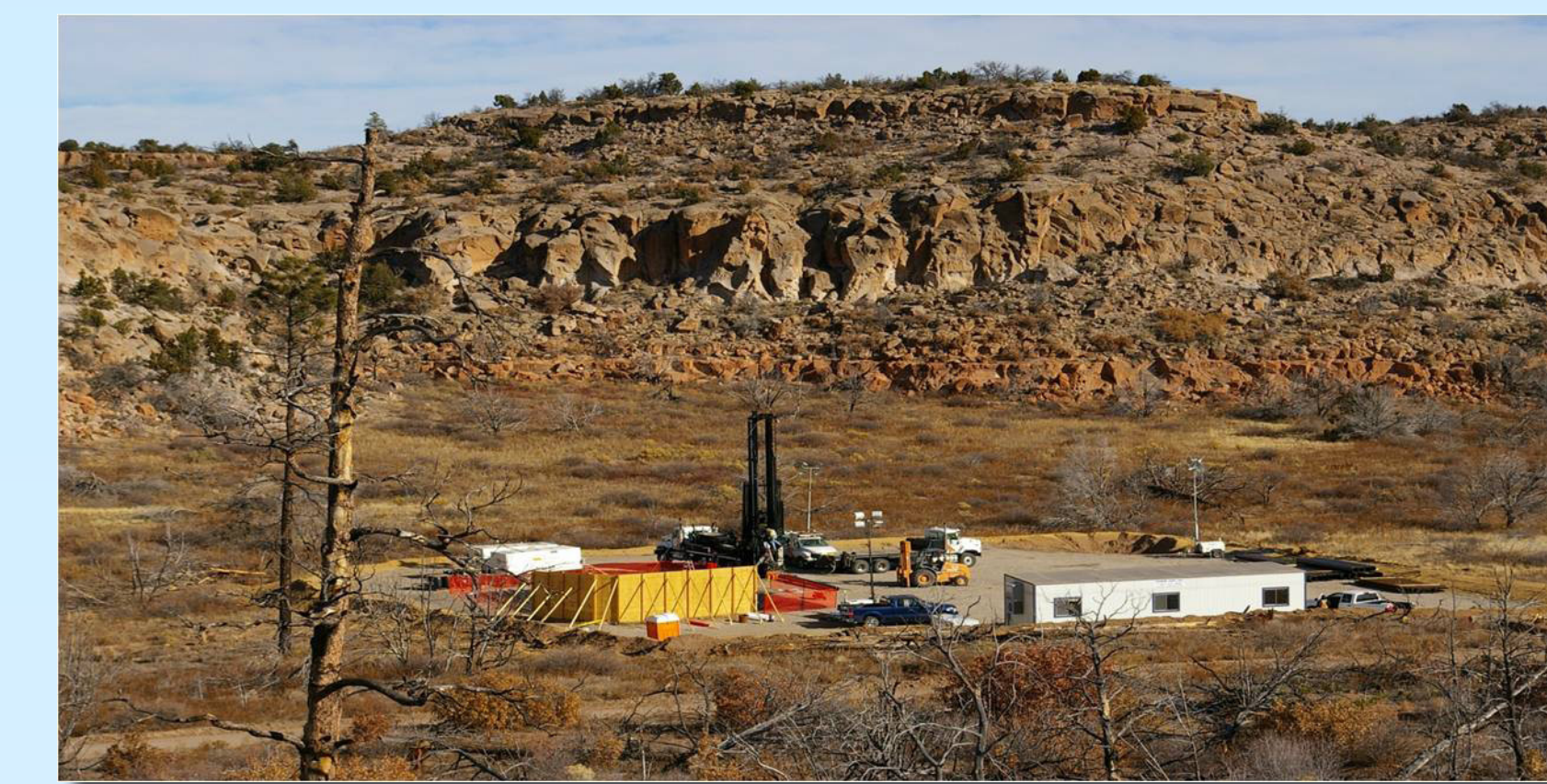
Regional Well Installation
