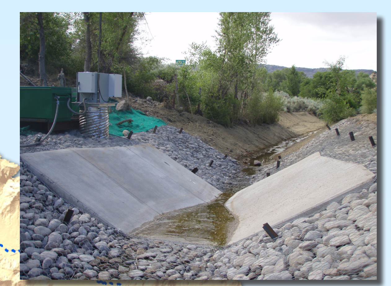
Gaging and sampling station. Measures flow.
