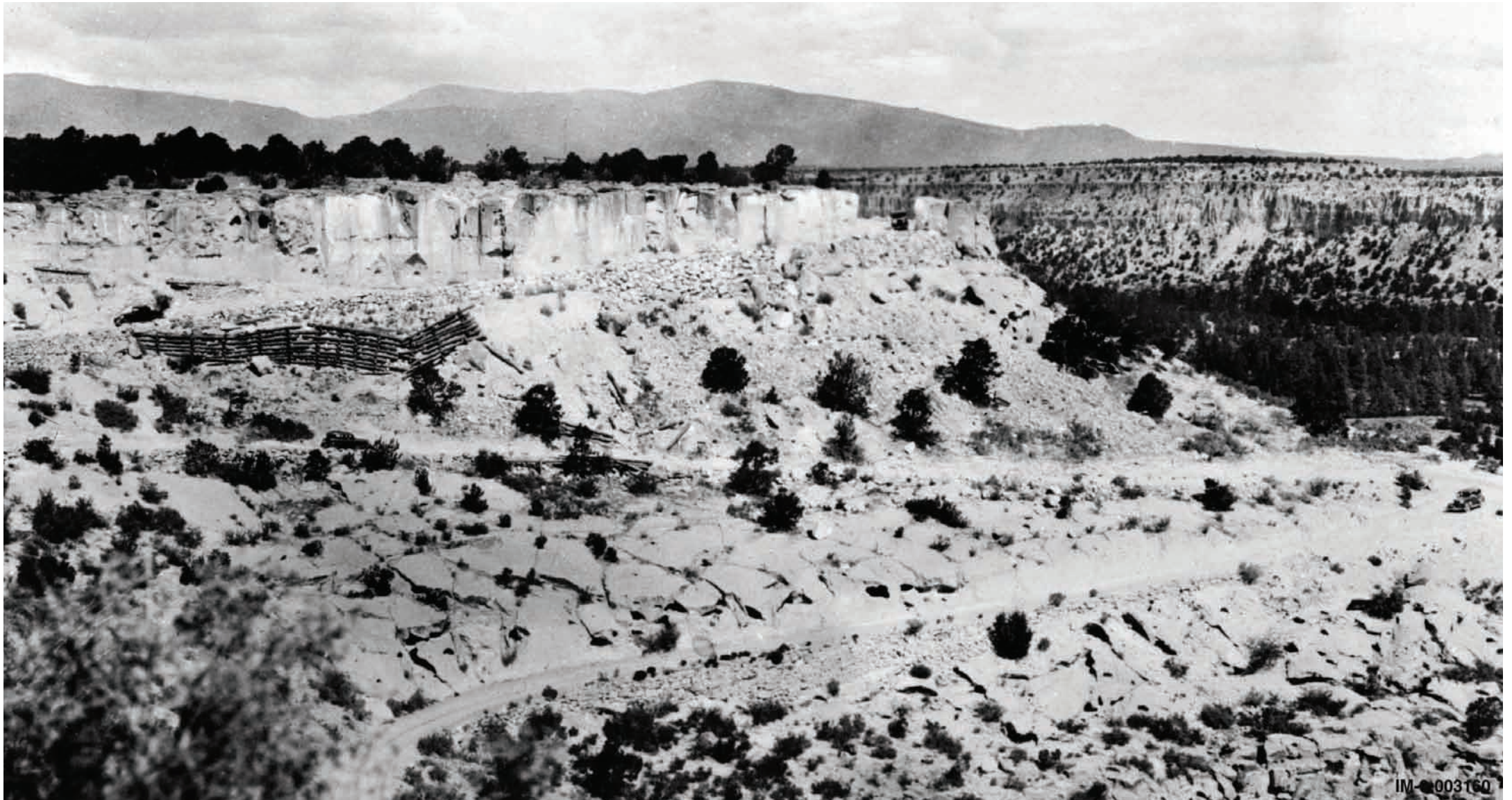
Figure 46. The original main road to Los Alamos challenged early automobile traffic. Large vehicles could not make the final, tight curve (compare this photo to photo on previous page) and had to back up the last section of the old dirt road. The Ranch School improved the road, bypassing the last switchback and extending it more gradually to the right, through the gap shown at the end of the mesa. (Los Alamos Historical Society)
