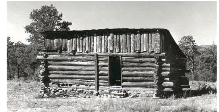
Figure 61. In contrast, the Romero cabin had a shed roof. (Los Alamos National Laboratory)
