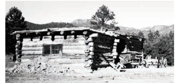
Figure 65. Close scrutiny of this 1942 photo reveals a shaded dog trot, or covered passageway, connecting the two ends of the Efrén Durán cabin. (Los Alamos National Laboratory)
