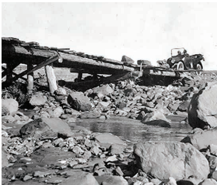
Figure 47. The lumberman Henry S. Buckman built this bridge across the Rio Grande, as well as a sawmill and a train siding. The bridge was the primary crossing to the Pajarito Plateau until 1921, when a new road bridge was built a little farther north at Otowi Crossing. (Los Alamos Historical Society)
