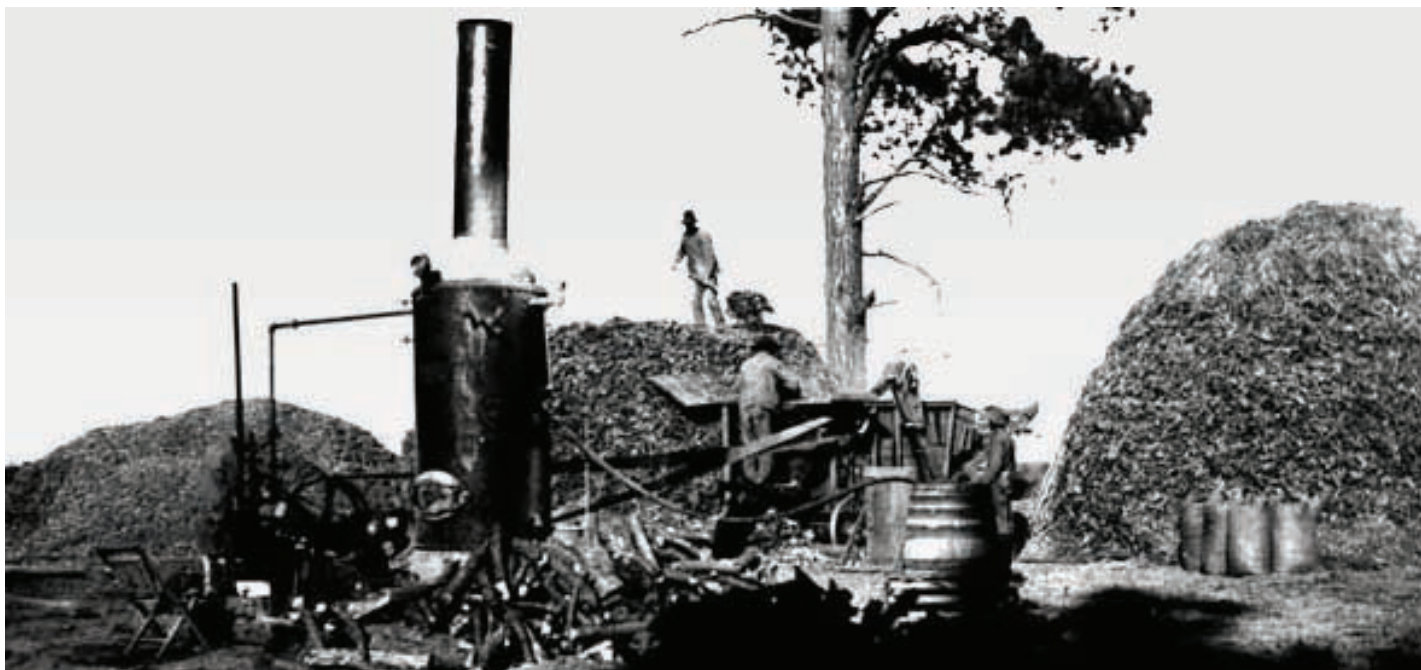
Figure 95 (first three photos). The equipment at the Ranch School included a reciprocating steam engine used to saw wood. The need for firewood for cooking and heating homes was constant on the Pajarito Plateau. The operator shown in top left photo is identified in the original caption as "Henry Cook, retired engineer on Santa Fe RR." Photo is dated 1922–23. (Los Alamos Historical Society)
