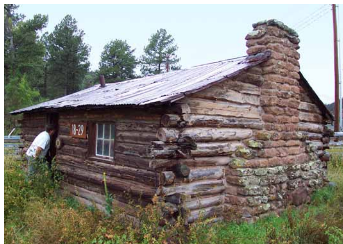
Figure 66. The Pond cabin in Pajarito Canyon, on the grounds of the Pajarito Club, featured a substantial stone fireplace and chimney. (Los Alamos National Laboratory)
