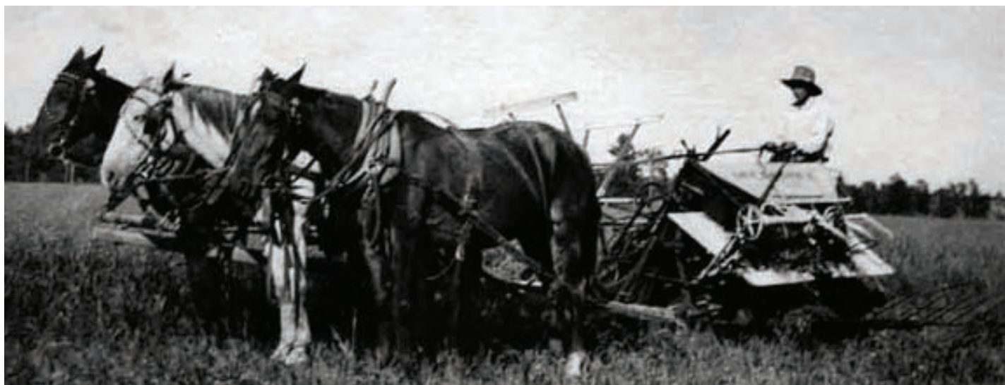
Figure 90. A team of horses pulls a twine binder on the plateau. Horse-drawn twine binders were first marketed in 1880 and were the chief method of harvesting grain on small holdings until the early twentieth century. The binder cut and bundled the grain. (Los Alamos Historical Society)
