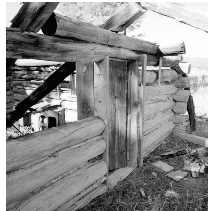
Figure 63. The spaces between the logs of the Miguel Sánchez cabin were chinked with small strips of wood. (Los Alamos National Laboratory)
