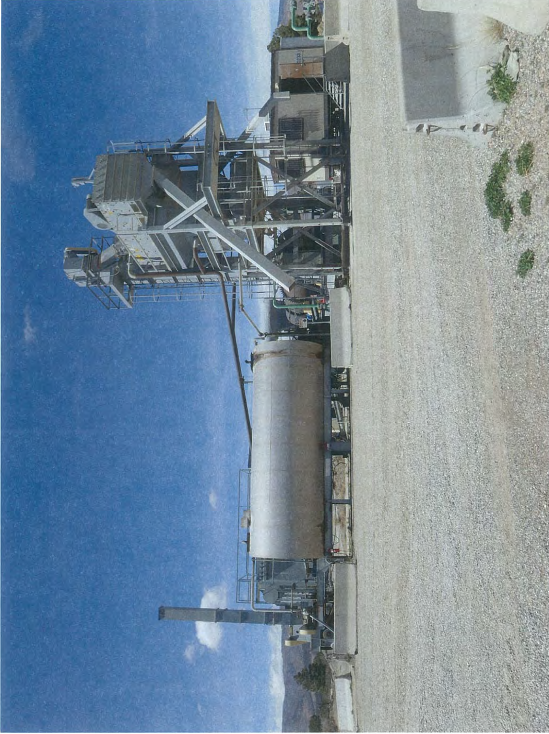
Photograph 1. Looking W towards the TA-60 ABP To the left is the 115 gal. oil tank. In the center is the 15,000 gal. asphalt cement tank. Secondary containment is located below these tanks.
