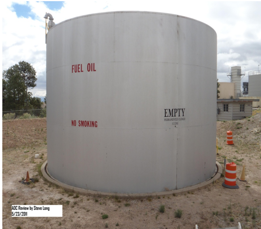
Photo 1. AST #26 (Emptied, Cleaned and Permanently Closed in Place as of May 2011)
