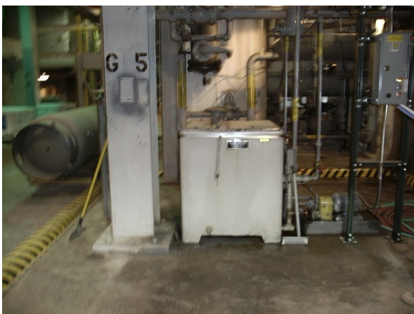
Photo 14. Oil Purification Unit in Bermed Area
