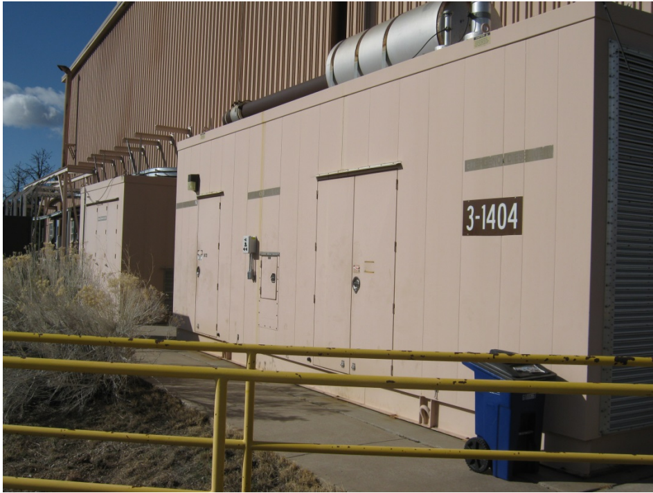
Photo 4. 1.25 MW Standby Generator (Structure 1404)
