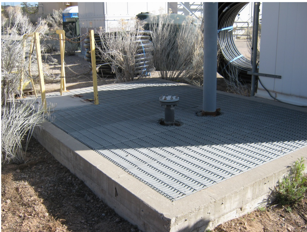
Photo 7. CGTG Oil/Water 2000 Gallon Below Grade Storage Tank With Secondary Containment TA-3-2305
