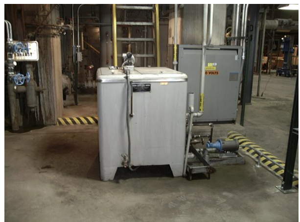
Photo 15. Oil Purification Unit in Bermed Area
