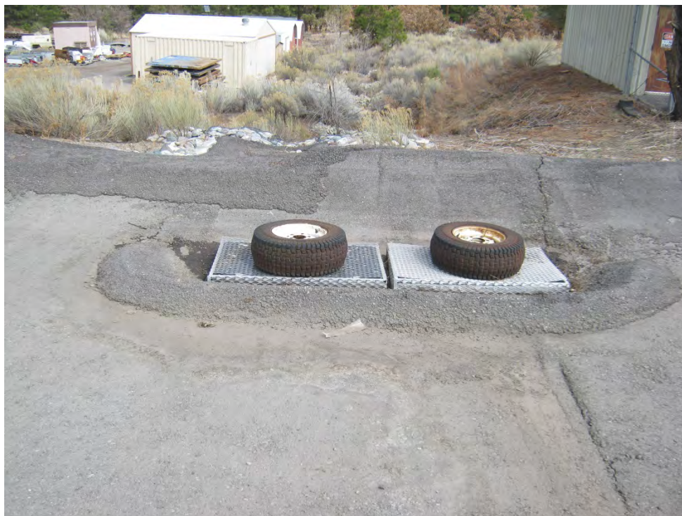
Figure 1: TA-60-1 parking area storm drains equipped with PetroBarriers™
