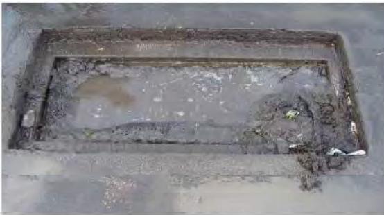
The water has been evacuated from the surrounding area by raising the overflow valve. Directly under the grate the mud, sludge and debris is removed.
