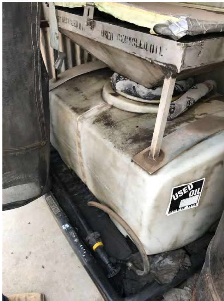
Photograph 2: 125-Gallon Used Oil Tank Located In Southeast Section of TA-60-1
