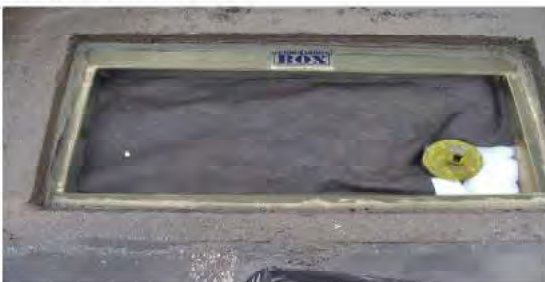
All of the dirt, mud and debris is cleaned from the pre-filter in the flanged area. New filters are installed above the Petro-Barrier-Box, none of the dirt made it through the filters.
