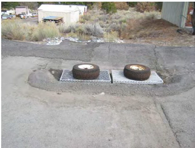
Photograph 10: TA-60-1 parking area storm drains equipped with PetroBarriers™
