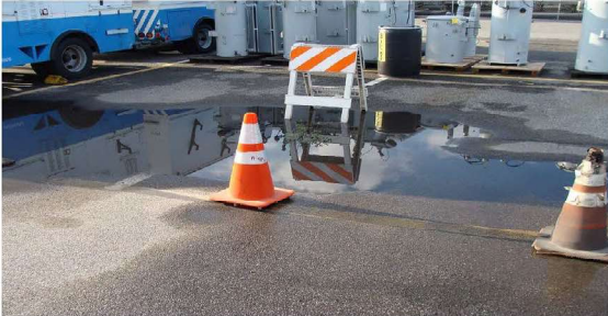
Water has backed up from the storm drain. Petro-Barrier-Box is not draining well and needs maintenance.
