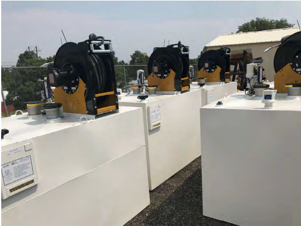
Photograph 8: 500-Gallon Oil Tanks for Hydraulic Oil and Motor Oil Storage At TA-60-1
