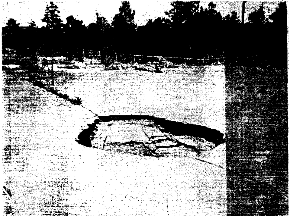
Figure 7.3-2 Appearance of the collapsed section of asphalt over Area 2 in 1975, viewed to the west. Hole area was about 3 ft by 6 ft and the depth was about 3 to 4 ft.
